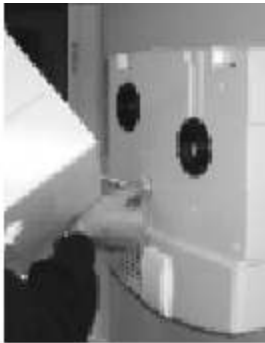
3. Attach the low voltage cable connector to the counter-piece of the filtering unit. The connector of the low-voltage cable is in a separate package.
