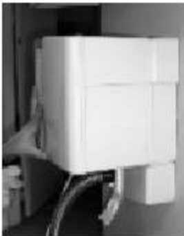
6. Set the central unit straight towards the filtering unit. Check that the rubber parts behind the unit coincide with the counter-pieces.
