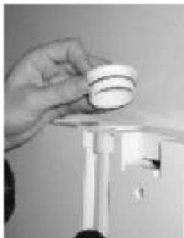
15. If additional wall inlets are added to the system the plug on the upper edge of the unit is to be removed. This allows to take additional wall inlets from the filtering unit, e.g. behind the wall or to the other rooms.
